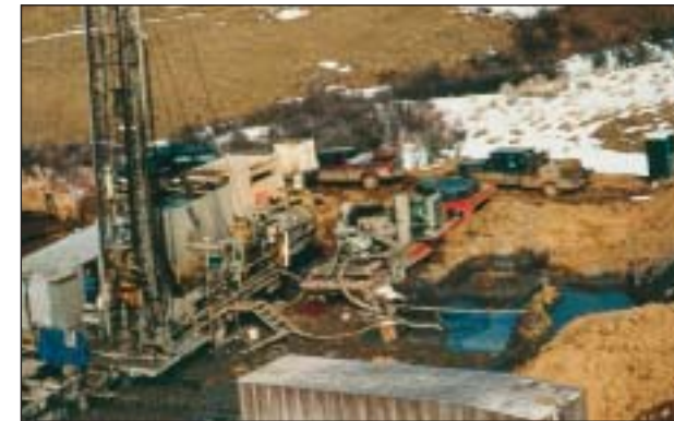
Coal bed methane gas drilling platform — POWDER RIVER BASIN RESOURCE COUNCIL
